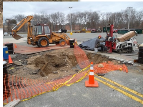
Installation of Groundwater Monitoring Wells Surrounding an Excavation
